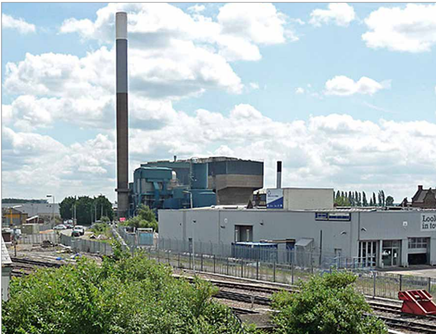
Figure 2: Eastcroft Incinerator in Nottingham (Source: © Stephen Richards [cc-by-sa/2.0])
