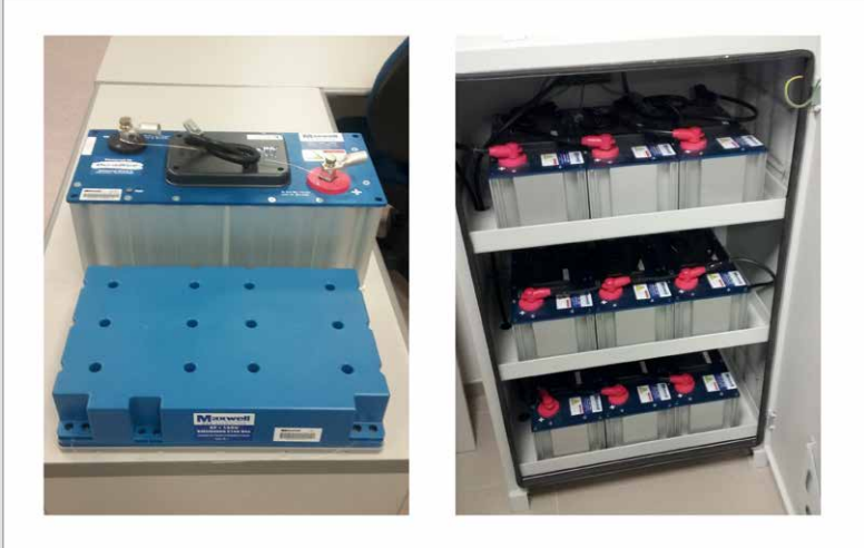
Figure 10: Ultracap close-up and rack with ultracaps (Source: ZIGOR Research & Development A.I.E).
