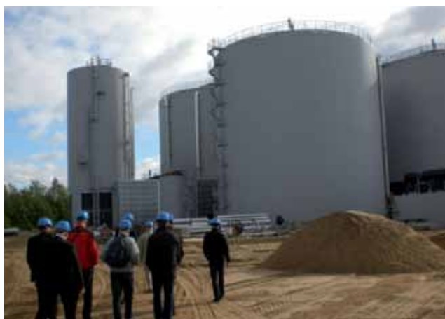
Image 5.2: Biogas Plant in Måbjerg (DK)
