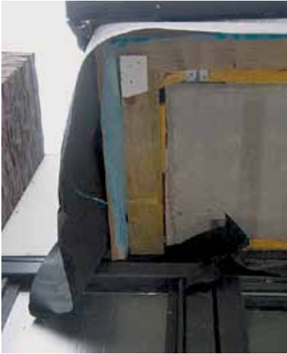
Image 2.1 External Wall Insulation in Almere (NL)
