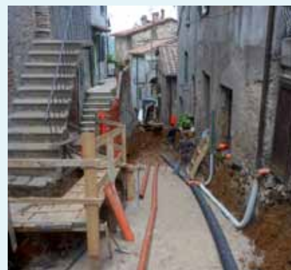
Image 3.6: Installing Geothermal District Heating in the Historic Centre of Montieri (IT)
