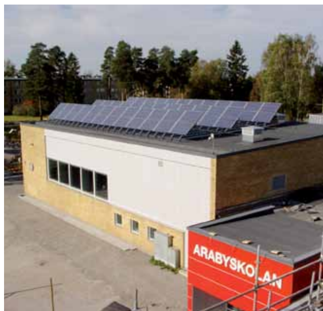
Image 4.2: The Araby School in Växjö (SE) is being Refurbished and a PV Plant is Installed on the Roof
